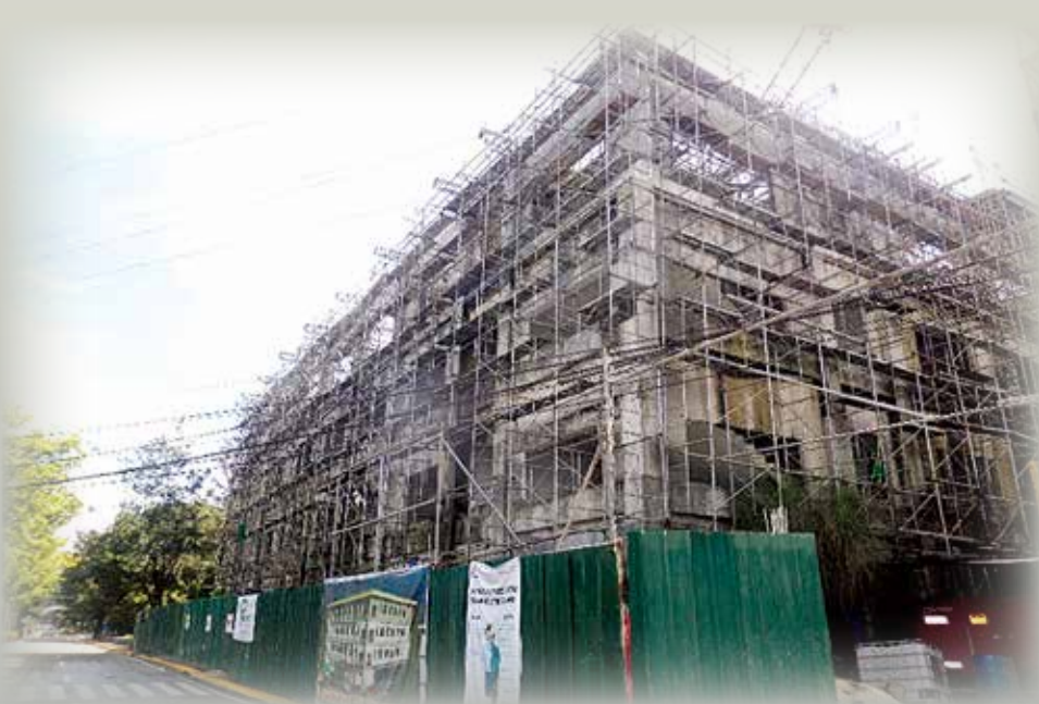
Construction of Four-Storey HAG and HTG Building
